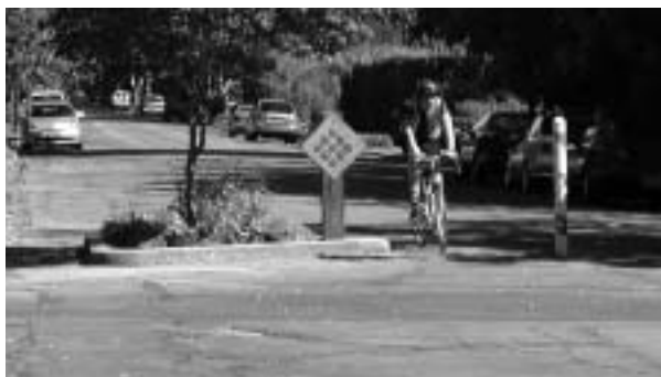
Traffic diverter on Bryant Street Bike Boulevard in Palo Alto. Bryant Street has been a bike boulevard for over 20 years. Residents love it and bicyclists find it a pleasant and safe route for riding the entire length of the city.
