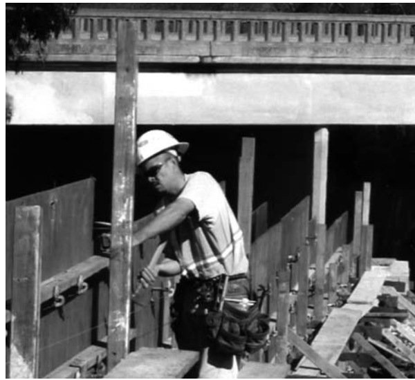
An extension of the river levee under Highway 1 will provide car-free access to the Tannery Arts Center, Harvey West, and the homeless shelter. It will allow cyclists heading into the San Lorenzo Valley to avoid the Highway 1 and 9 intersection. Thanks to the city Redevelopment Agency and Public Works, who have kept the project on track despite many challenges. Come appreciate their work at a ribbon cutting ceremony in April (exact date will be posted when available on peoplepowersc.org .)
